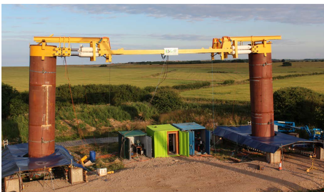
2.0 m diameter pile testing at Cowden in the UK
