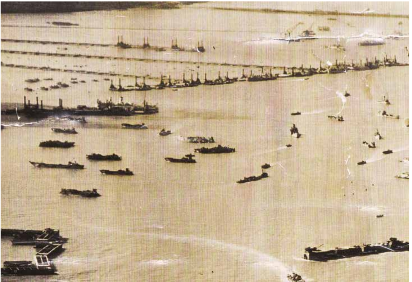
Aerial view of the British Mulberry in operation (image taken by A.R.W. Adcock, Tom Adcock's grandfather, who worked on the harbours' design and construction)
