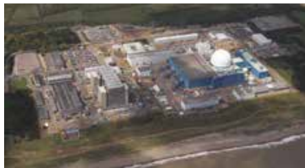
Sizewell B nuclear power station
