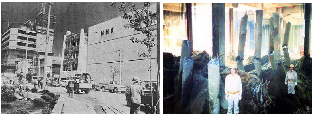
Figure 2.24: NHK Building suffered damage to its pile foundations during 1964 Niigata earthquake and tilted 76^\circ on its long span. But, the damage pattern of pile was observed only after being excavated 20 years after the earthquake (Tazoh, 2007).
