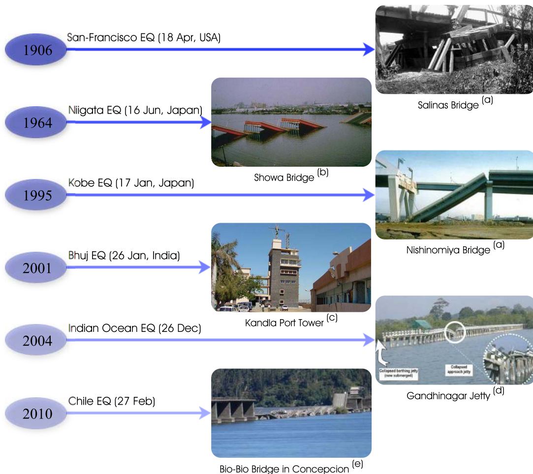
Figure 1.3: Failure of pile foundations during various earthquakes. (Sources: a) NISEE (2010), b) NGDC (2010), c) NICEE (2010), d) Mondal & Rai (2008), e) Photo by Daniella Escribano L.)
