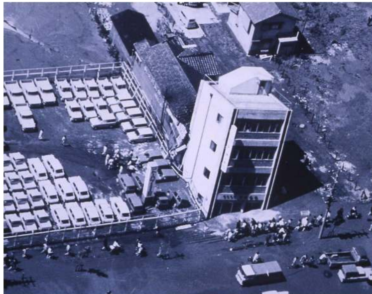
Figure 1.1: A building leaning due to liquefaction of subsoil near Niigata Station during the 1964 Niigata earthquake (JGS, 1964).
