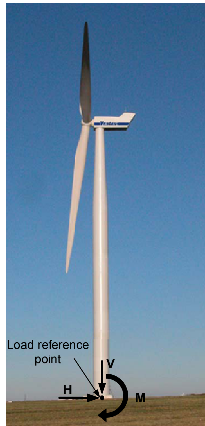
Figure 1.2.10. Photograph of wind turbine with assumed loads shown acting at the base of the tower. (Vestas (2004))
