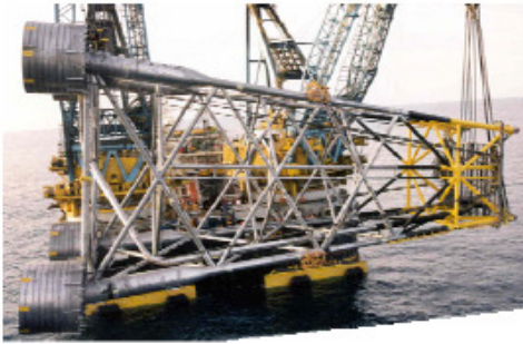
Figure 1.1.1. The Draupner jacket showing the 12 m diameter caisson foundations at the base of each leg. (Statoil)
